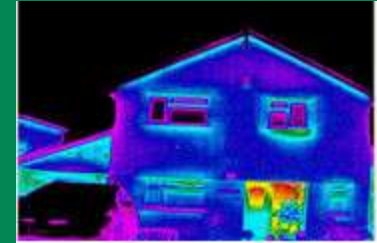
Thermal image of a home with insulation
