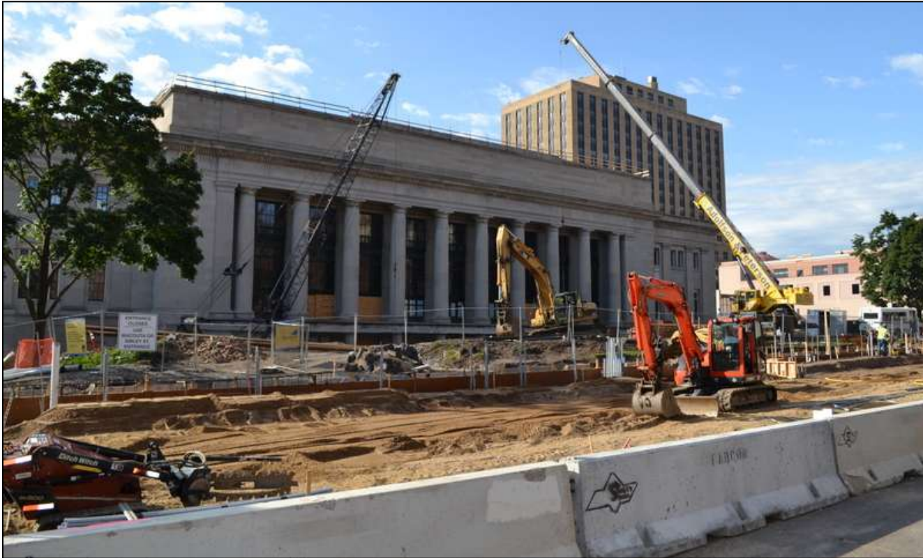
Plaza and light rail platform construction.
