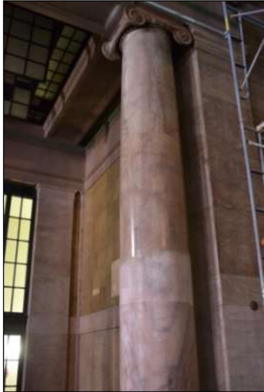
Marble column cleaning.
